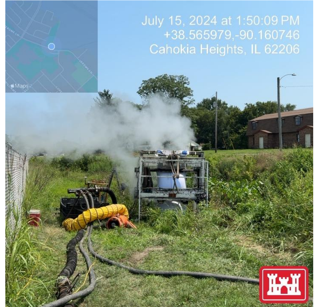
Curing Liner with Steam
